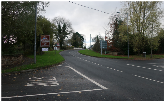
Public Road no. 206 of 208, Muff, Co. Donegal.
